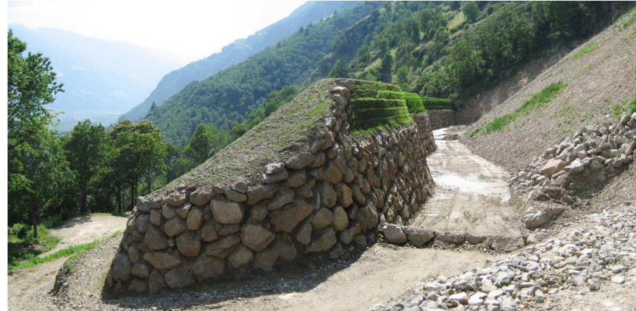
Rockfall retaining wall ( www.ingph.eu )
