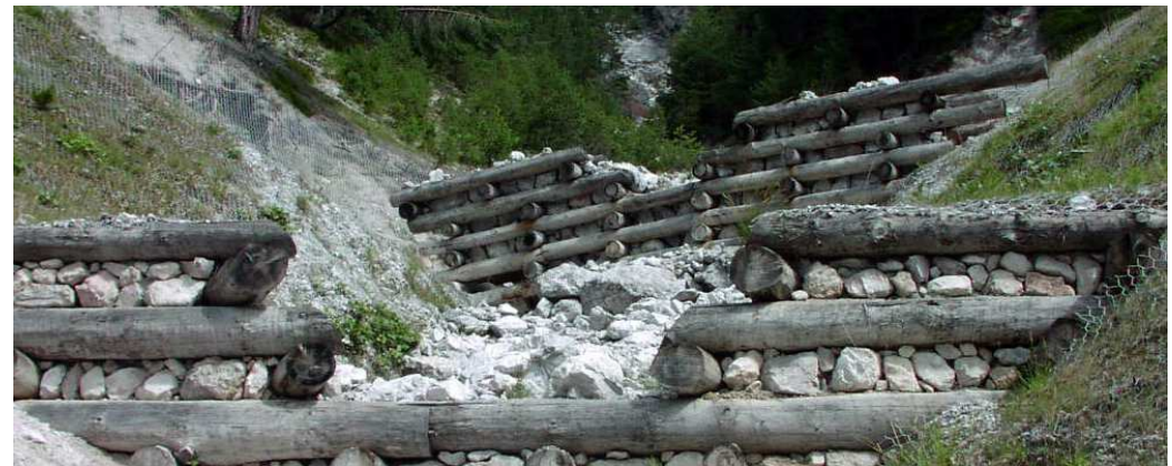
Consolidation check-dams (Foto Studio Archeng)
