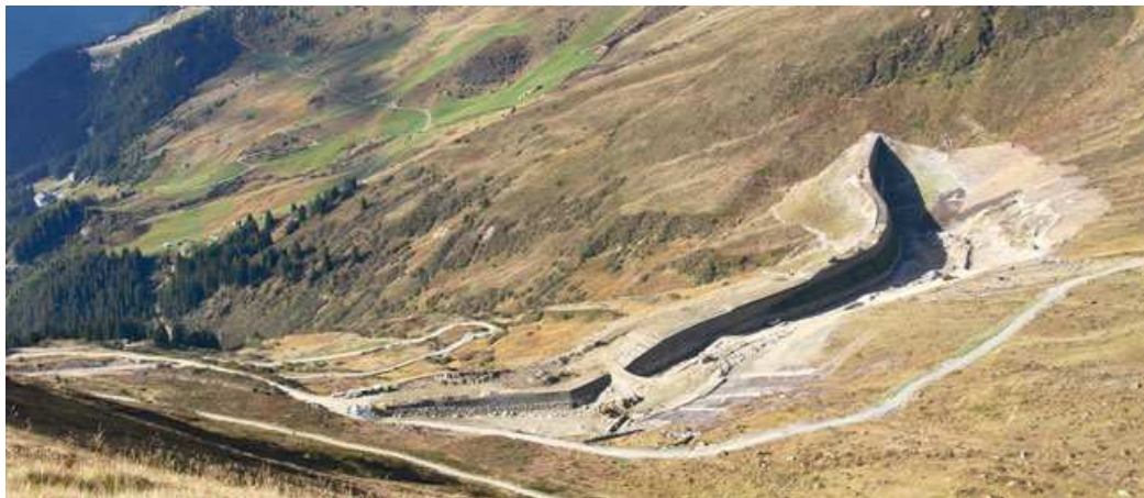
Avalanche retention barrier ( www.eagm.eu )
